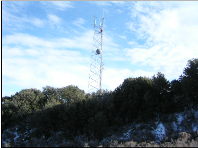
Photograph 3: Overview toward Santiago Peak candidate location, facing west.
